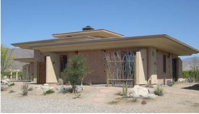
Fig. 5: Well Designed With Large Overhangs and Minimal Glazing
