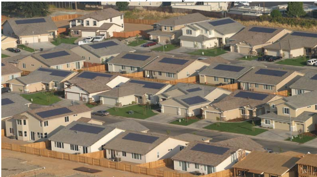
Figure 1. Premier Gardens ZEH Community: 95 Highly Energy-Efficient Homes with 2 kW (AC) Solar Systems
