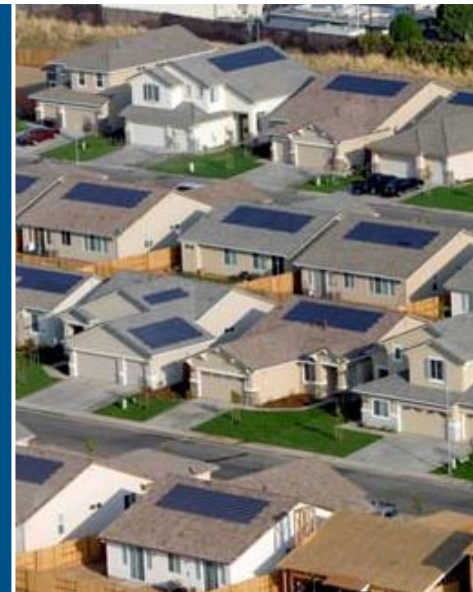
A view of the 95 homes of Premier Gardens, all today's zero energy. Photo courtesy of Sacramento Municipal Utility District.
