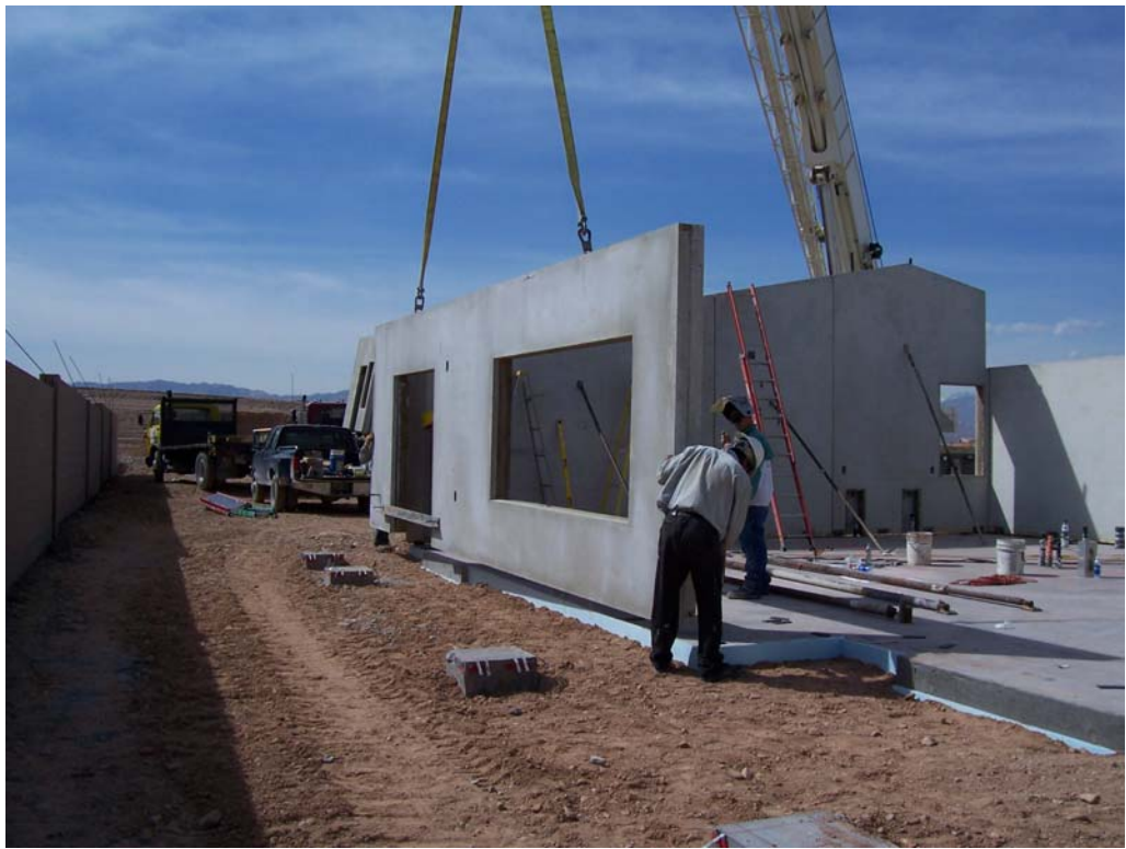
Figure 6. The erection of the T-Mass walls for the Zero Energy House.
