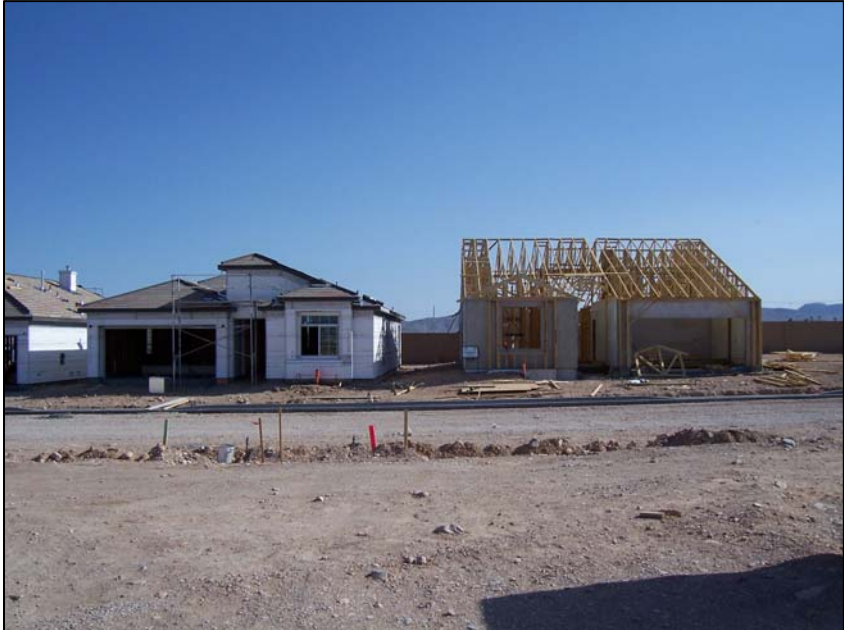
Figure 3 Wood frame house on the left and T-Mass on the right.
