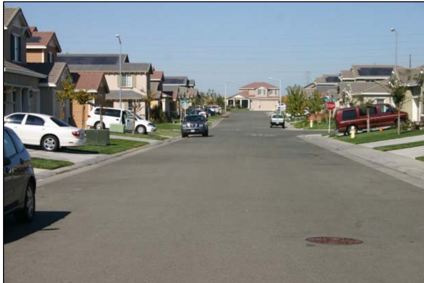
Figure 8- Solar Roofs at Premier Oaks
