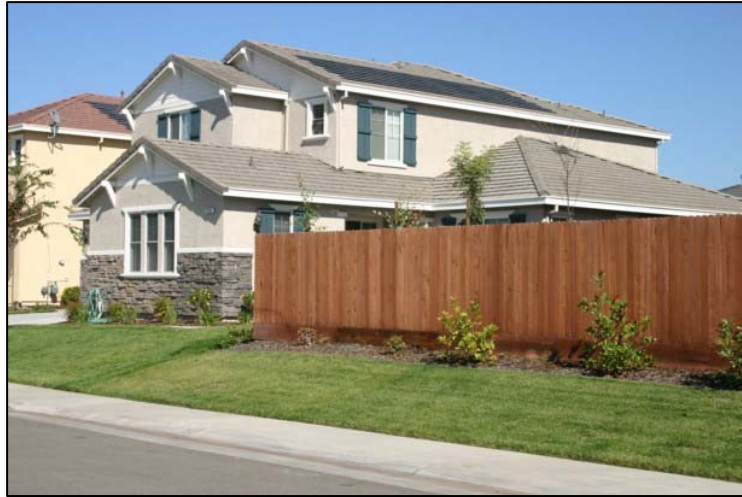
Figure 7- Integrated 2.4 kW PV at Premier Oaks
