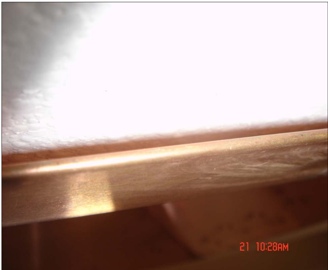
Figure 8: Close-up View of Skylight Perimeter
