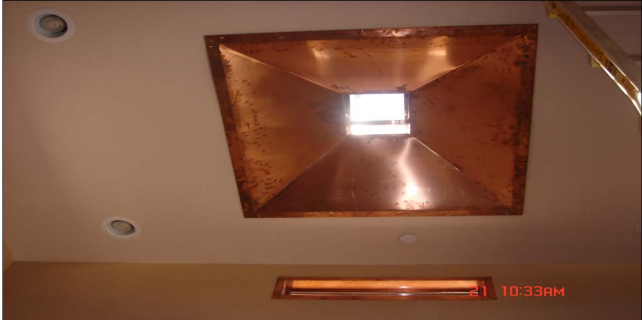
Figure 6: Example Custom, Site Built Ceiling Skylight Penetrations
