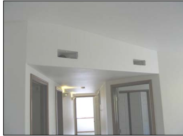
Figure 6 Condict ductwork located within conditioned space, pre- and post-drywall
