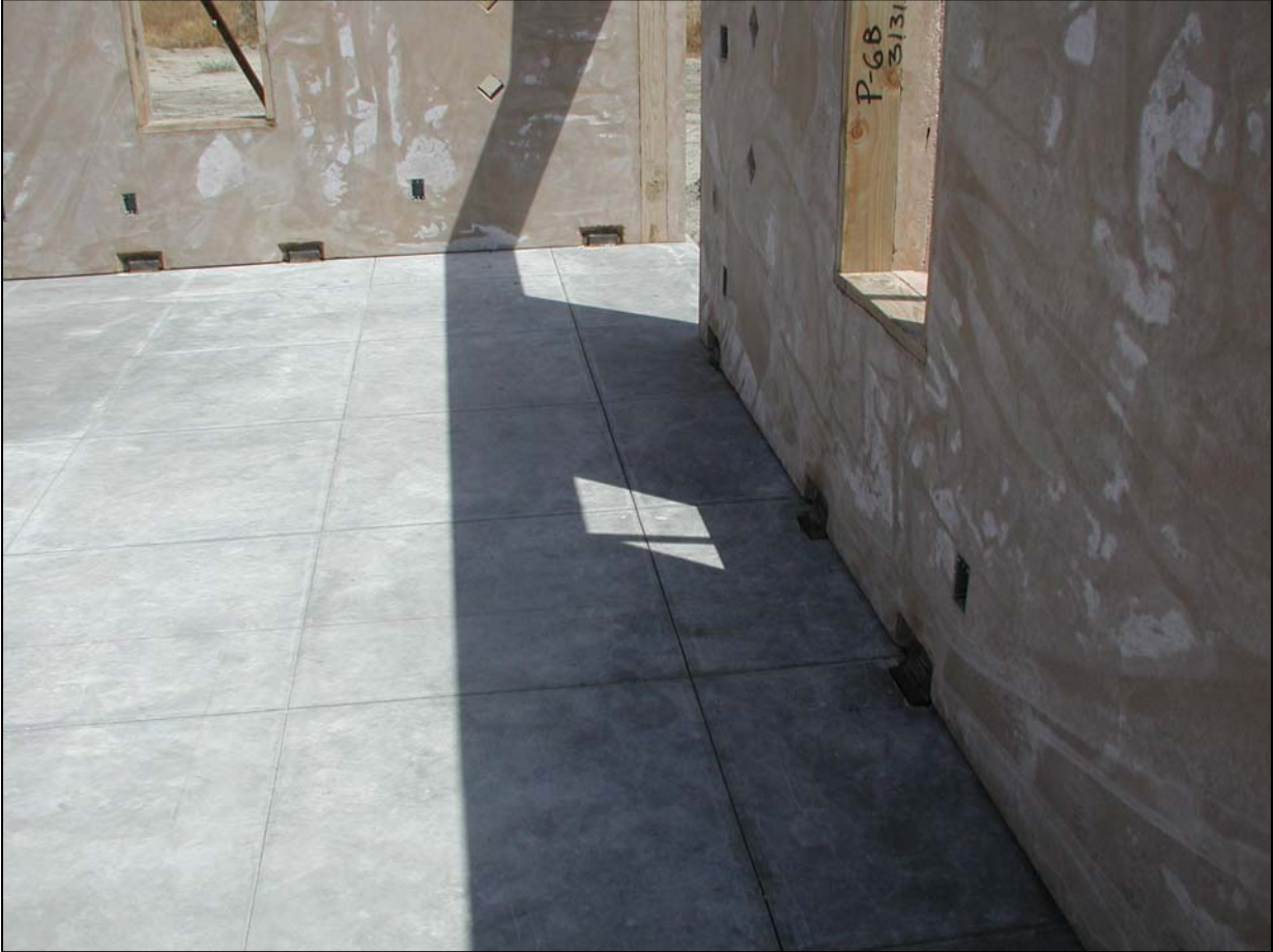
Figure 15: T-MASS ® Weld plate on floor
