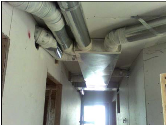
Figure 6 Condict ductwork located within conditioned space, pre- and post-drywall
