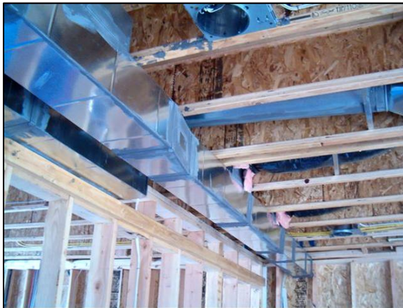
Figure 7 New Traditions Ductwork, pre- and post-drywall
