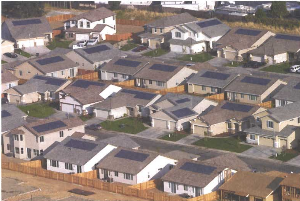
The PV systems in the Premier Gardens ZEHs are supplying approximately 50% of the electricity used in the home—an average of 3,333 kWh annually, out of the total average of 7,007 kWh consumed.
