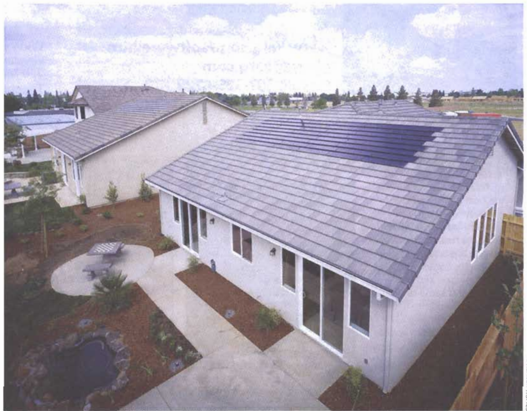
Premier Gardens is a 95-unit infill project designed for entry level first-time homebuyers. Roof-integrated PV panels (RIPV) are standard.
