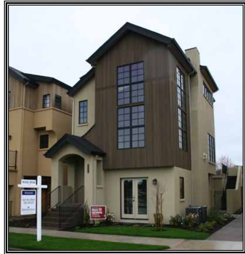
Building America Home featuring Solar DHW (Ruhoff Homes, OR)
