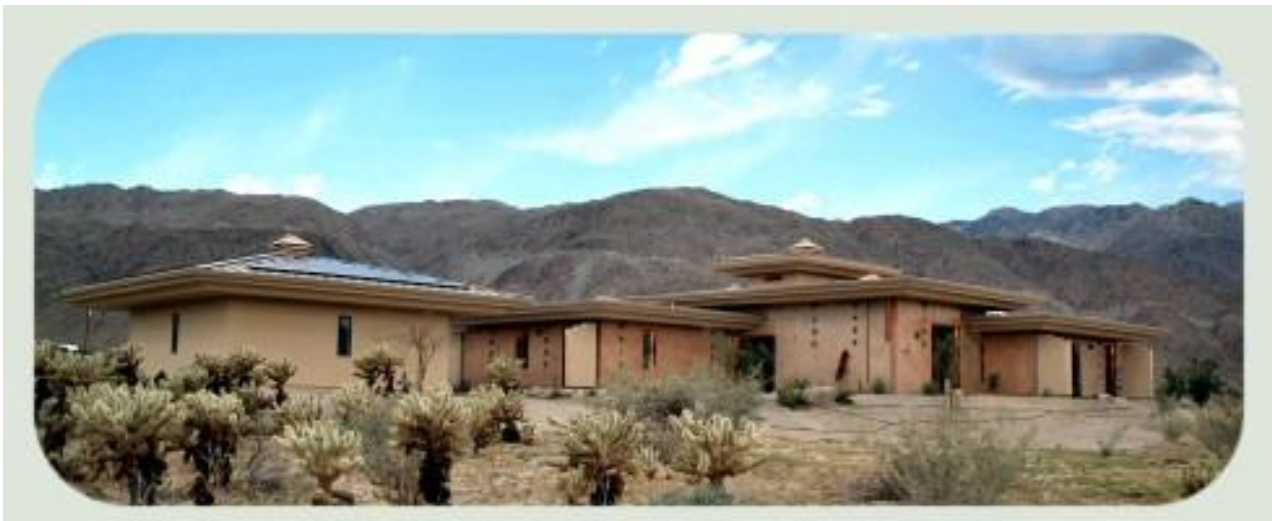
Figure 2: One of Four Borrego Springs Prototype Houses
