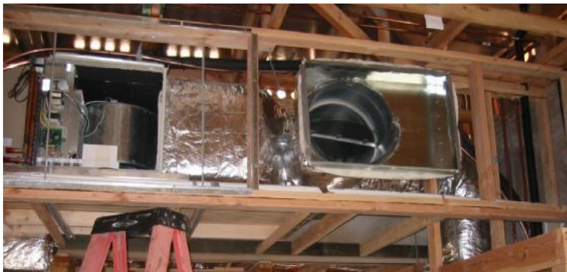
Figure 17: NightBreeze Air Handler and Damper Installation, DiGiorgio Site
