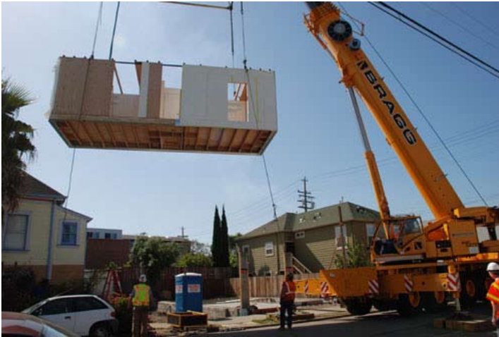
ZETA delivers modular home to construction site
