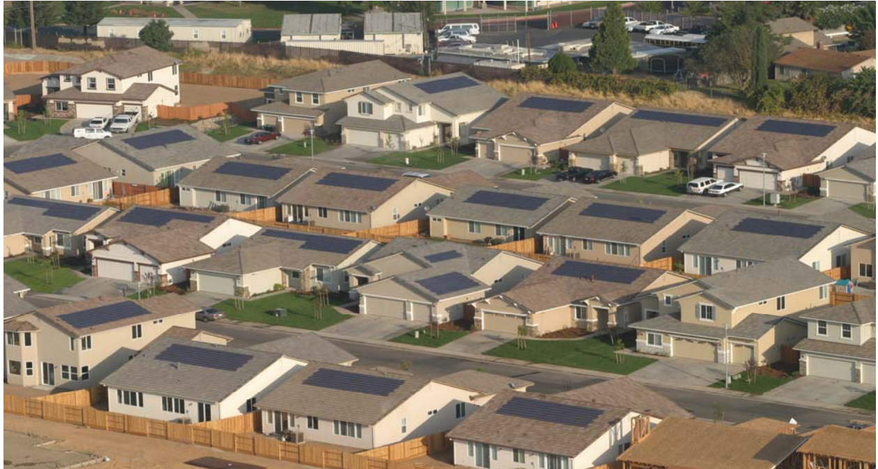
Fig. 2: Premier Gardens community showing PV systems on roofs (courtesy of GE).
